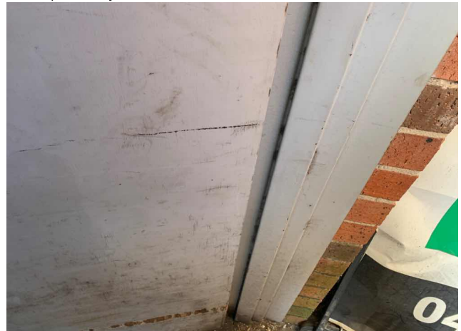
2.1 - External / GF / Perimeter / Doors and door frames / Topcoat -Blue (J220192255LP1.7) - <0.1%w/w
