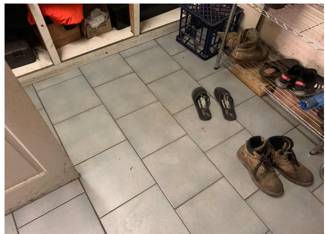
34 - Internal / GF / Staff changing room / Beneath the ceramic tiles / (J220192255NA1.3) - Presumed to contain asbestos or hazardous materials
