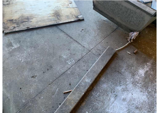
41 - Internal / GF / Warehouse / Expansion joints within concrete / Bitumen (J220192255A3.1) - NAD,ORG
