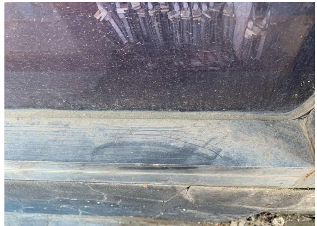
5.1 - External / GF / Perimeter / Reception step and stonework / Topcoat - Black (J220192255LP5) - 0.14%w/w
