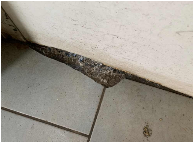
9.1 - Internal / GF / Kitchen / Beneath ceramic tiles / (J220192255La1.1) - Presumed to contain asbestos or hazardous materials
