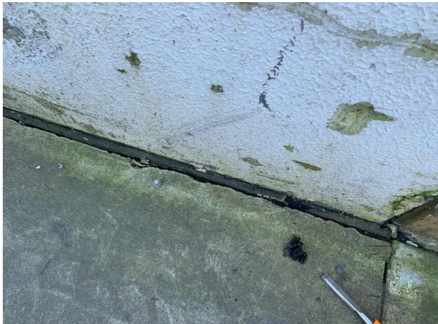
1 - External / GF / Perimeter / Damp proof course to walls and expansion joints / Bitumen (J220192255A3) - NAD,ORG
