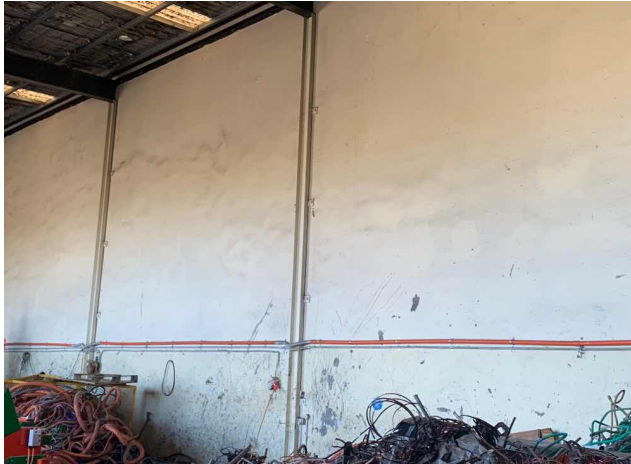
40 - Internal / GF / Warehouse / Concrete walls / Topcoat - Cream (J220192255LP2.8) - <0.1%w/w
