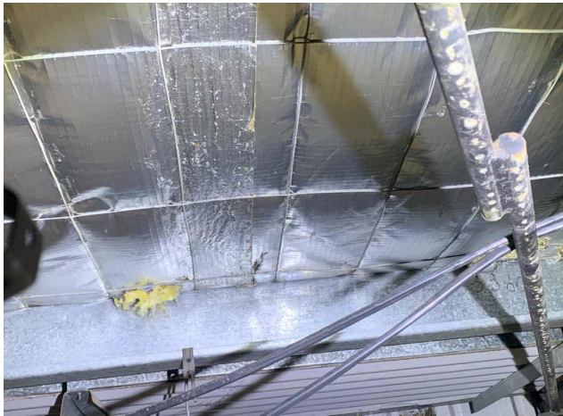
28 - Internal / GF / Roof void / Ceiling / Sarking Insulation (J220192255S1) -
