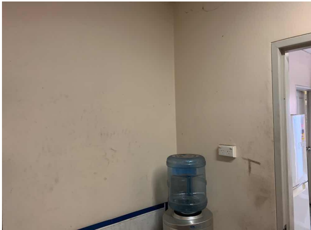
35 - Internal / GF / Staff changing room / Concrete walls / Topcoat -Cream (J220192255LP2.5) - <0.1%w/w
