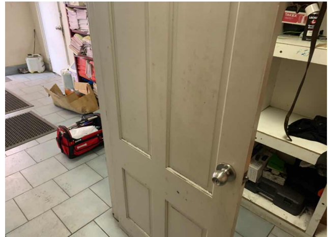
36 - Internal / GF / Staff changing room / Door and door frame / Topcoat -Blue (J220192255LP1.4) - <0.1%w/w
